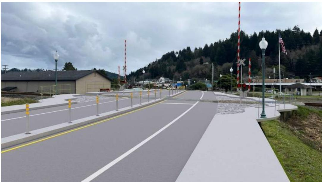
**Planning level cost opinion:** An order-of-magnitude planning level cost opinion was prepared for the median barrier on OR 38 based on unit costs from similar projects in the Pacific Northwest. The cost opinion accounts for design and construction along with several other factors. Potential right-of-way and property costs are not included at this time. The cost opinion is \$550,000.
